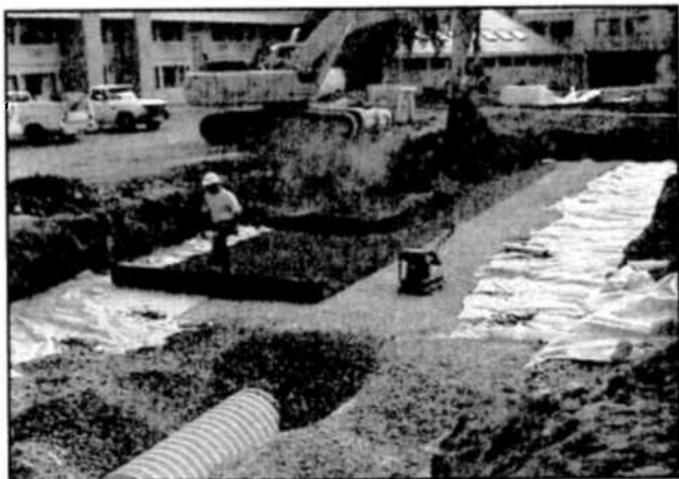
Roll out filter fabric.
