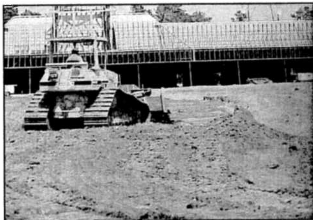
Continue to backfill the chamber bed.
