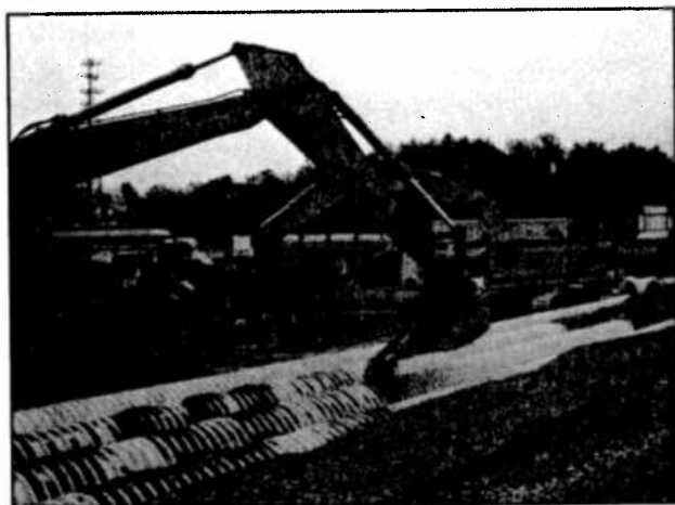
Carefully ladle 3/4 – 2 inch washed, crushed, angular stone over the centerline of the chamber row.
