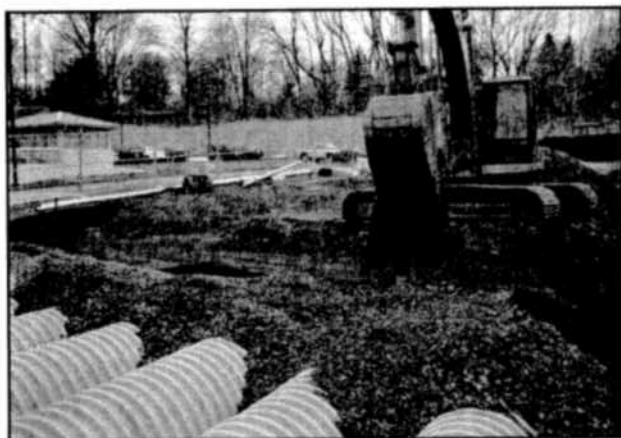
Backfill the bed using an acceptable fill material.
