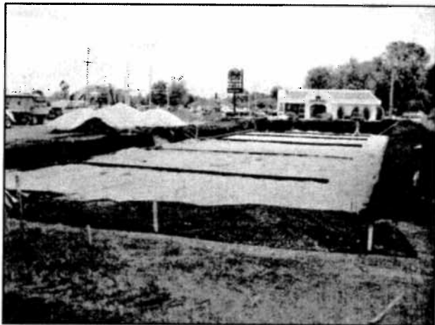
Filter fabric and underdrains installed.
