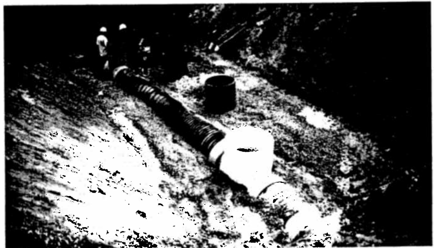
Backfill over the Water Quality Unit and installation of bypass line complete
