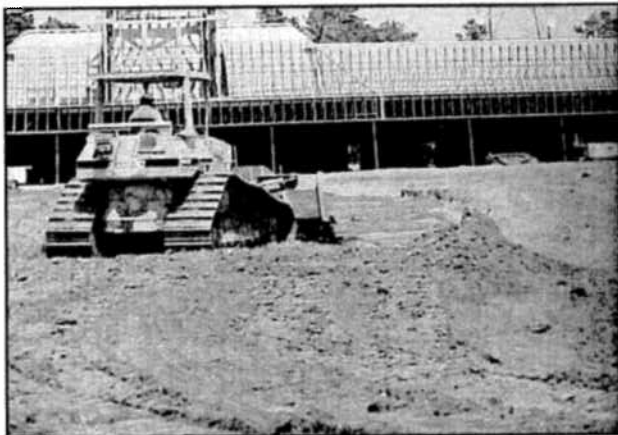
Continue to backfill the chamber bed.
