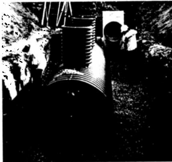
Setting the Water Quality Unit and the inlet tee fitting
