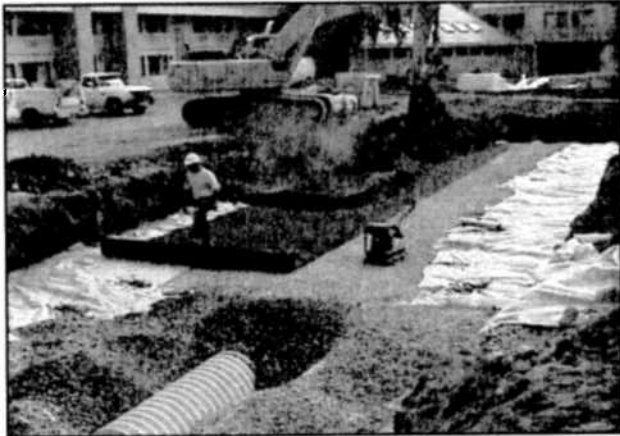
Roll out filter fabric.
