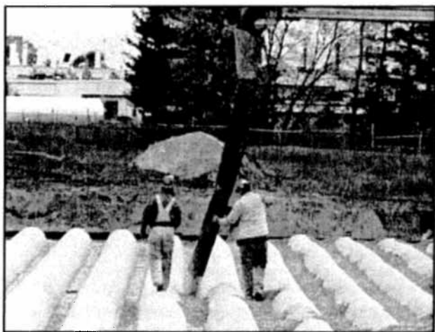
Evenly distributing stone with conveyor boom.
