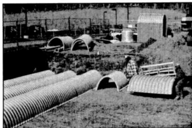
Maintain a minimum of 6" between chamber feet.
